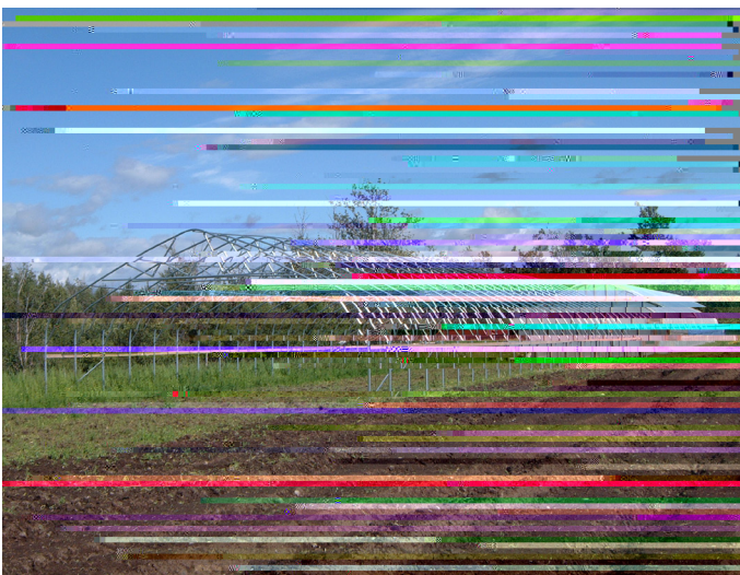
High tunnels have bent-pipe frames that are constructed of metal or PVC.
